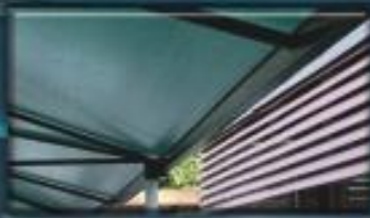
photo 3 Rectangular tubing surround on car port
