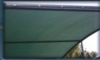
photo 4 Securing method using flat bar rolled in DriZ
